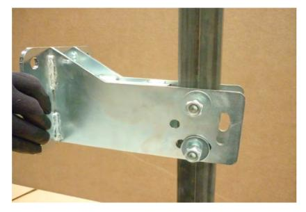
PLACE ROD INTO ROD HOLDER AND FIX WITH SCREW, NUTS AND BOLTS ASSEMBLY POSITION FOR ROD HOLDER DEPENDS ON INSTALLATION STUDY AND DESIGN
